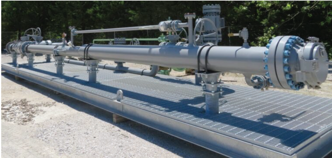
Figure 2. Pipeline trap.
