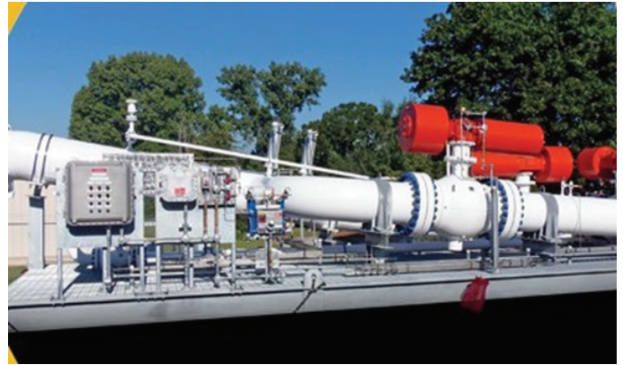
Figure 4. Pipeline trap components.
